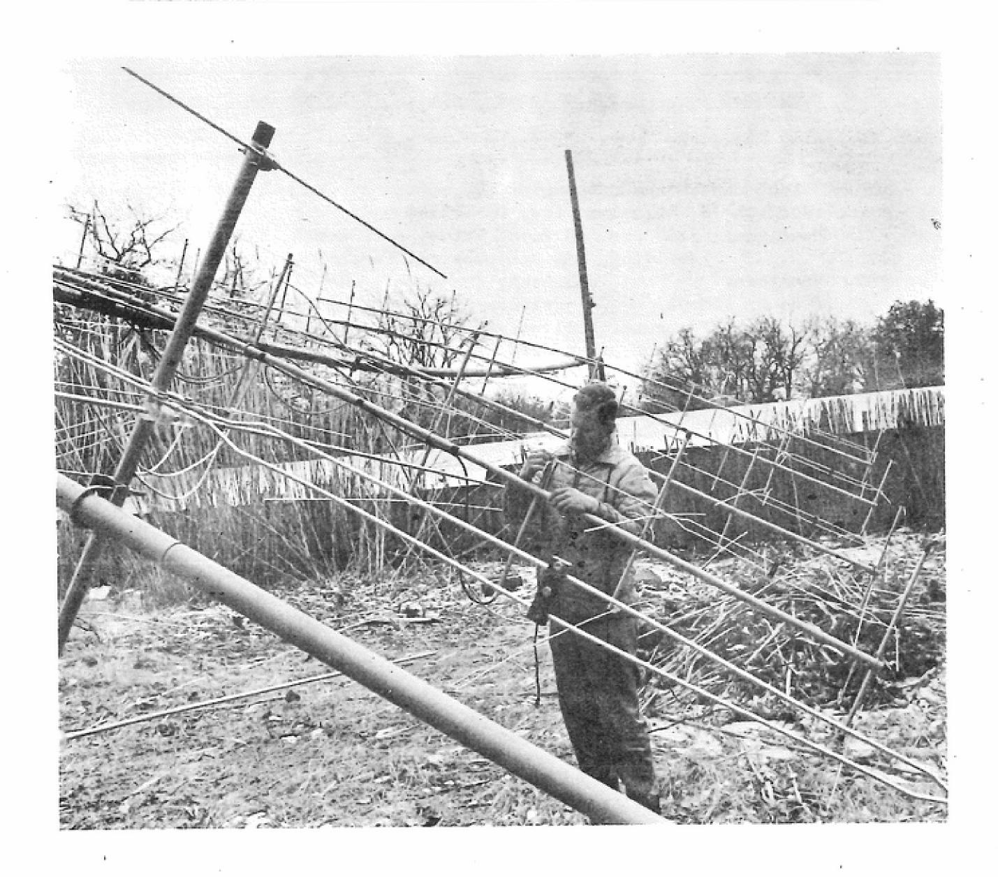
Marshall Williams, WASUNL, makes final adjustments on his 240-element antenna for 2-meter moon-bounce. For more details about the antenna, the largest of its type in the world, see story on page 17 (Photo by WA4AQW)
